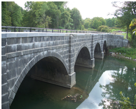
Aqueduct taking the Erie Canal over Nine Mile Creek
